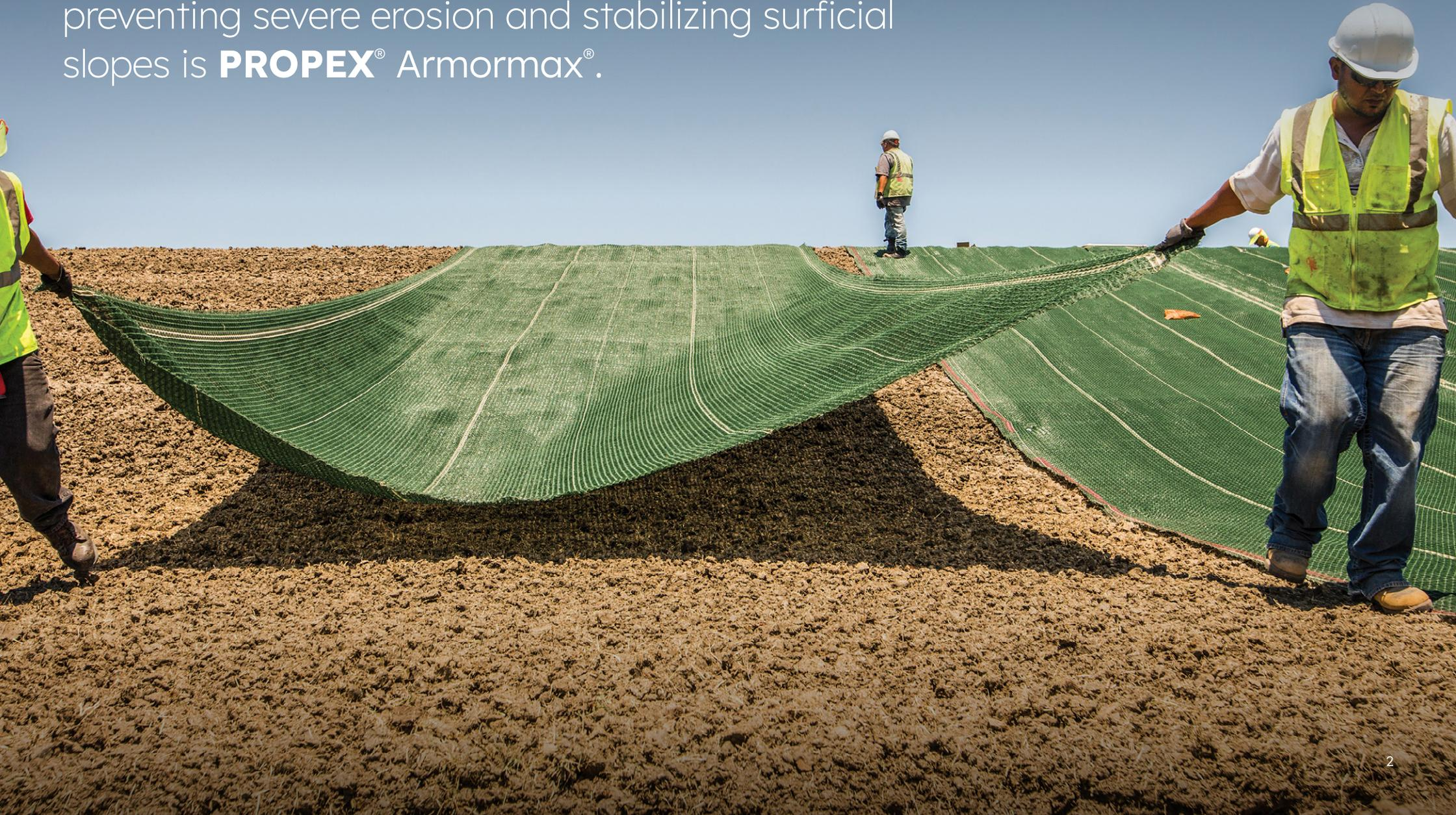
**PROPEX Armormax is composed of High Performance Turf Reinforcement Mat (HPTRM) and Engineered Earth Anchors that work together to lock soil in place and protect against hydraulic stresses.**
