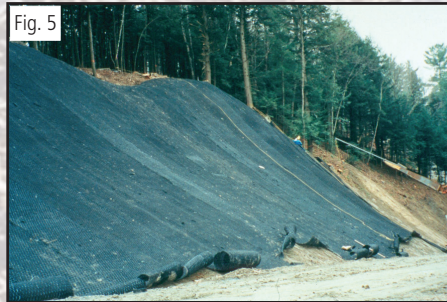
After installation and before vegetation
