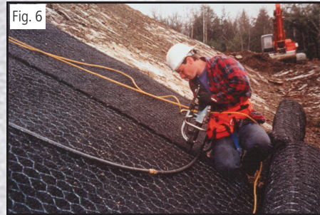
Adjacent MacMat® R panels connected using "hog rings"
