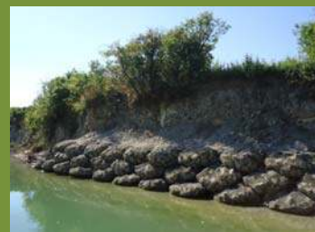
Czech Republic 2013 bank protection
