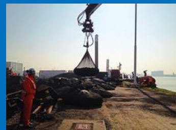
Belgium 2014 scour protection
