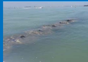
Italy 2009 create canal dike
