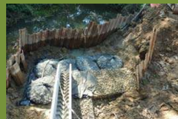
U.K. 2014 foot protection with gabion
