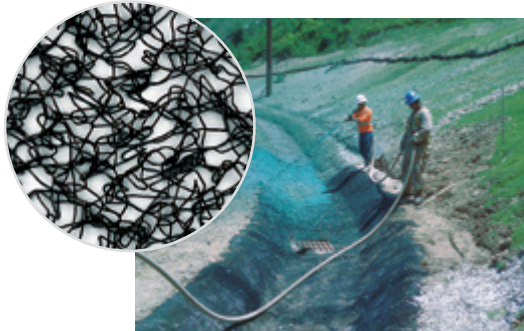
Slope interceptor ditch on steep slopes
