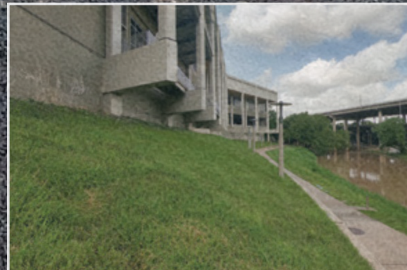
Three months after installation, thriving vegetation withstood flooding from Tropical Storm Imelda.
