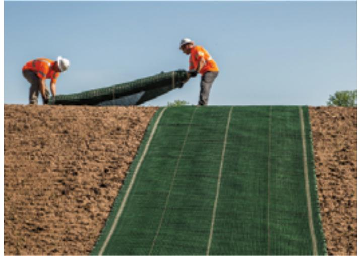
**HPTRM Laydown:** Unroll the HPTRM on the prepared soil ensuring material has intimate contact with the soil.
