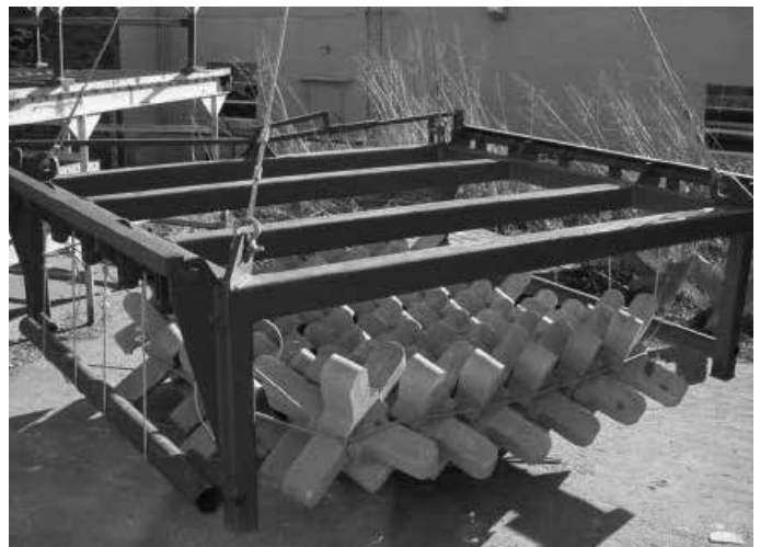
A cable must be run under every row of units to ensure the load is evenly distributed.
