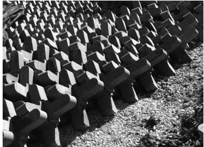
A-Jacks articulating concrete blocks (ACB) units should be placed on a bedding layer.
