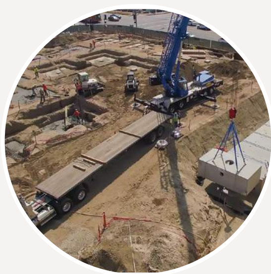
Same-day staging and installation.
