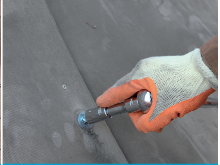
CC fixed to slope using rock bolt
