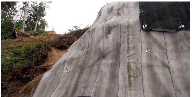
CC Slope Protection and Stabilisation project, Karapiro Gully, New Zealand
