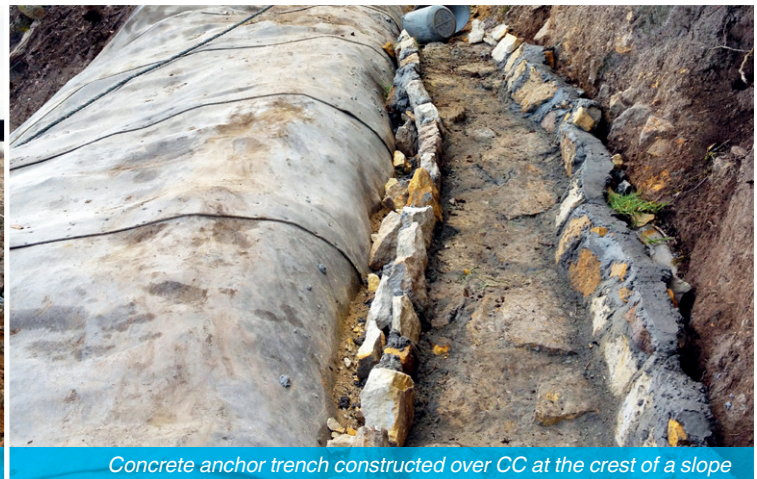
CC fixed at the crest of a slope with ground pegs and anchor trench
