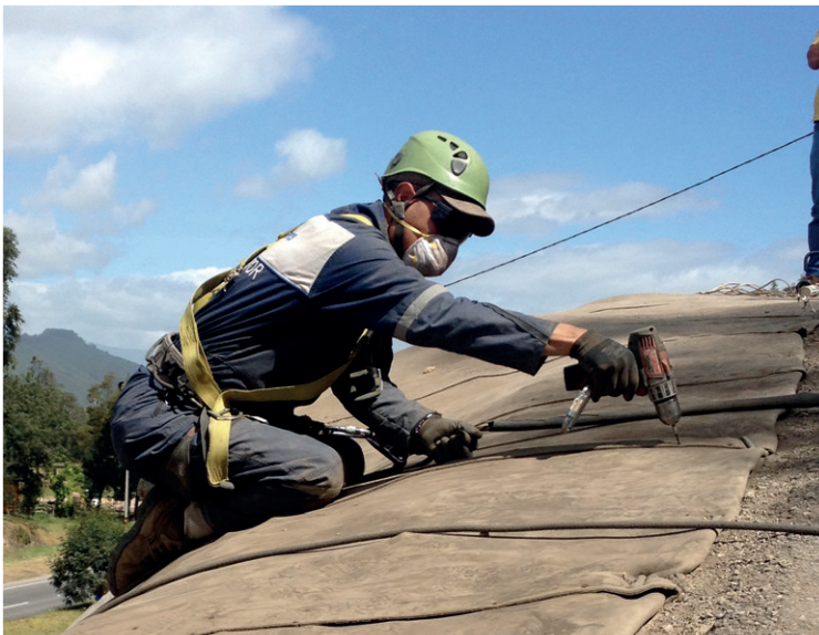
Jointing adjacent layers of CC using stainless steel screws
