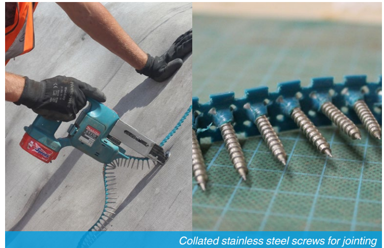
Mechanical fixings for connection to concrete
