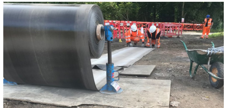
Bulk Rolls can be suspended from oil drum jacks and batched on site
