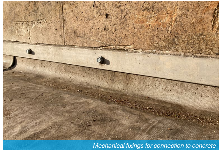
Typical J pegs for anchor trench edge fixings
