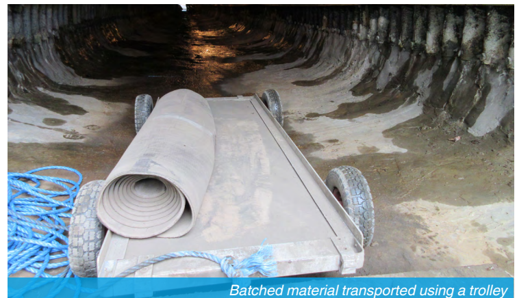
Bespoke batched CC transported into culvert
