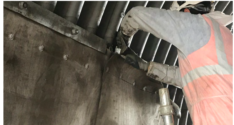
CC perimeter edge secured with clamping bar
