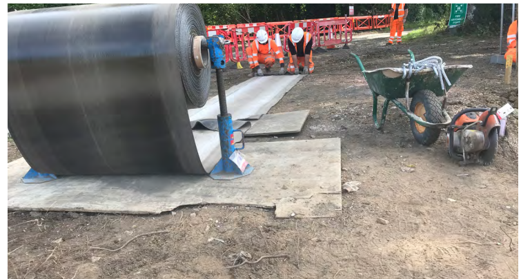
On site bespoke batching from a CC Bulk Roll
