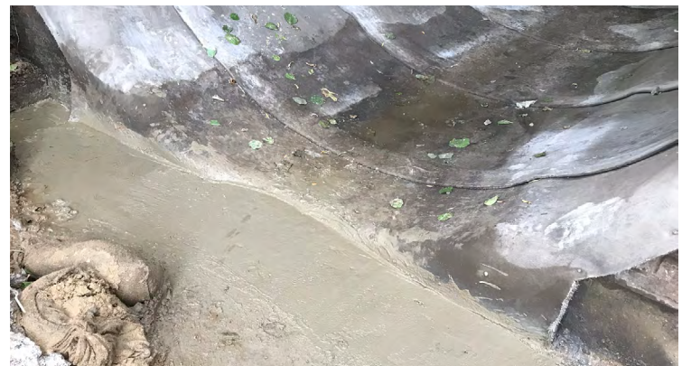
Leading edge buried in anchor trench
