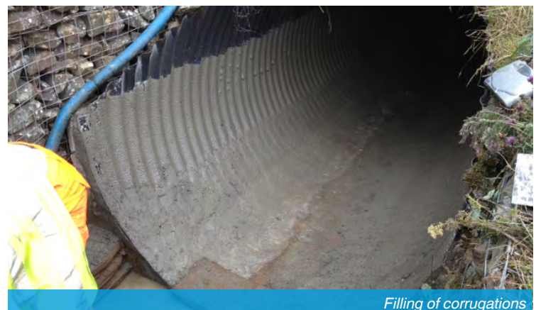
Smoothing over protrusions using grout
