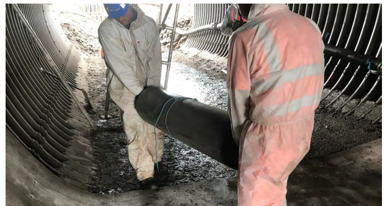
Bespoke batched CC transported into culvert
