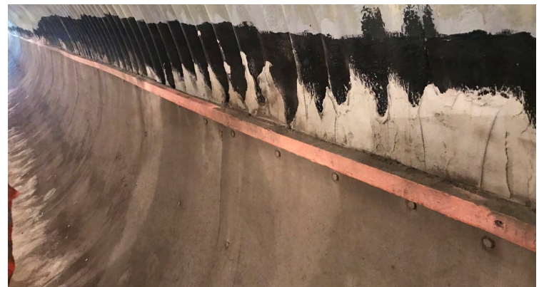
Timber secured to provide a cutting edge guide for a neat finish
