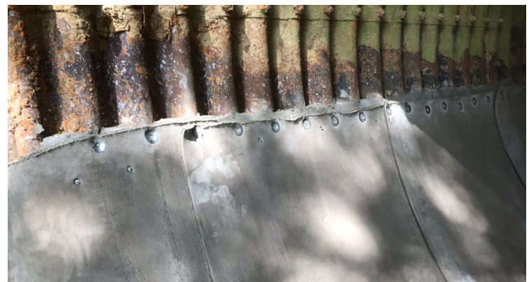
Perimeter edge secured with anchor fasteners and washers
