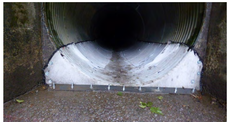
Trailing edge secured to concrete apron
