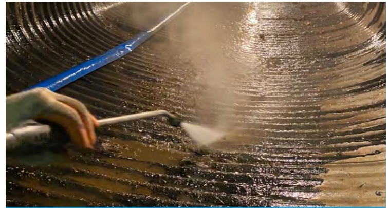
Power hose used to remove coatings and debris
