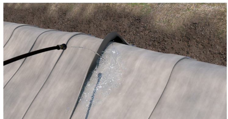
Hydration Under Joints Before Fixing
