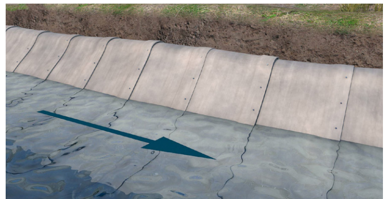
Overlap in Direction of Water Flow
