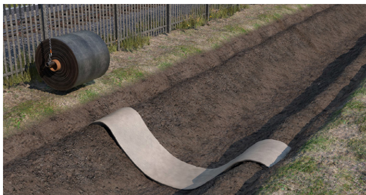
CC tucked into anchor trench prior to cutting
