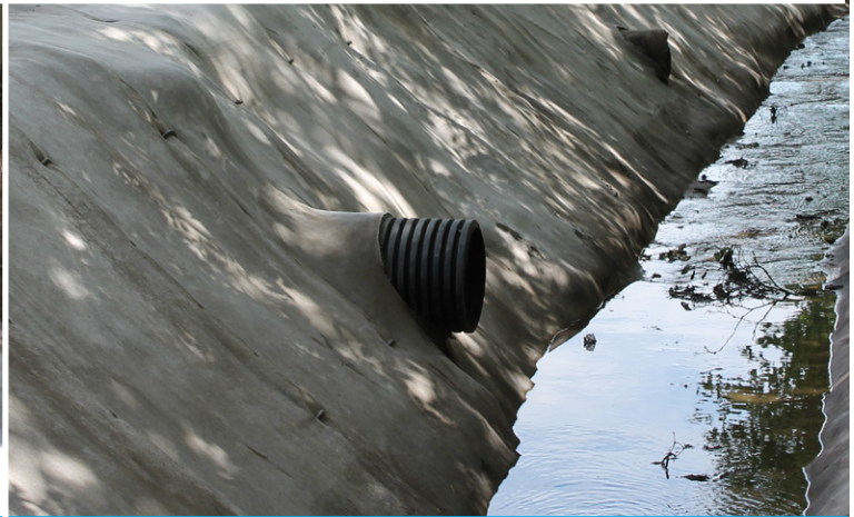
Retrospective pipe penetration
