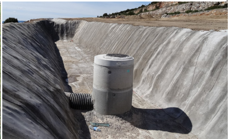
CC can be installed around existing infrastructure
