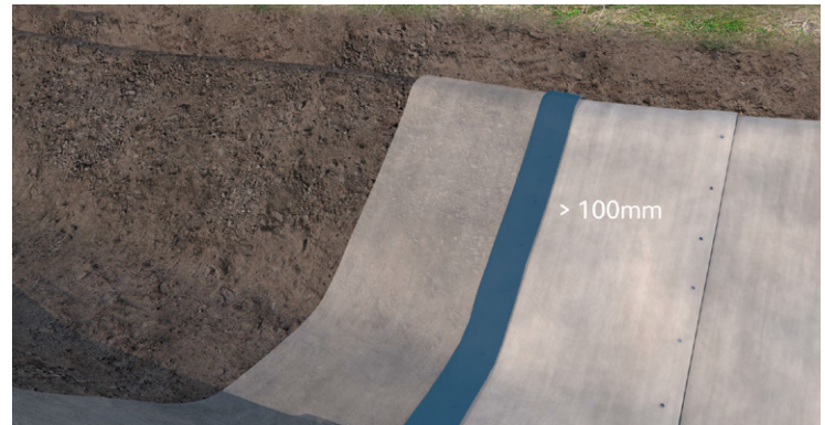
Overlap CC Layers by a minimum of 100mm
