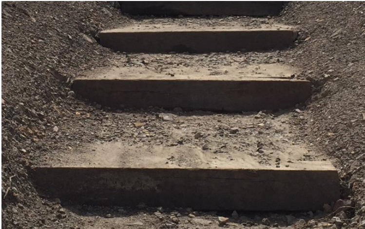
Baffles can be formed by laying CC over fabricated wooden structures or sandbags
