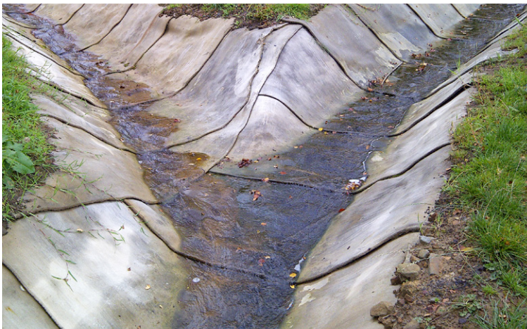
CC can be easily manipulated to form ditch junctions and terminals
