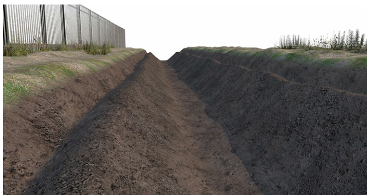
Substrate preparation & anchor trench
