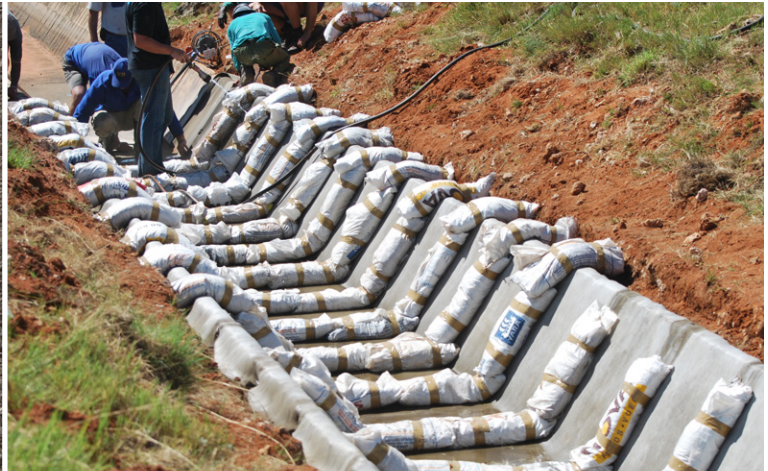
Sand bags can be used to compress joints during setting
