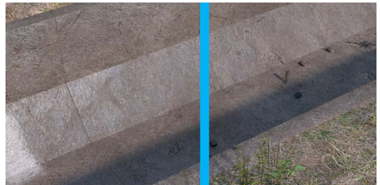
Failing mortar must be cleaned and mortar applied to large cracks
