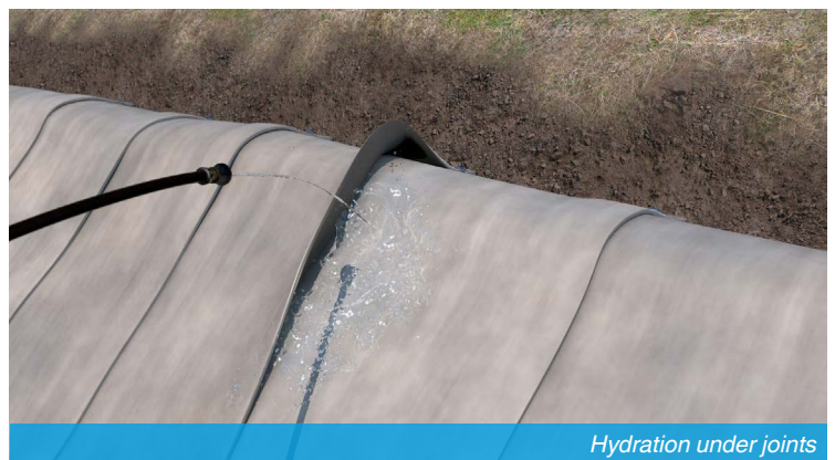
Overlap in direction of water flow
