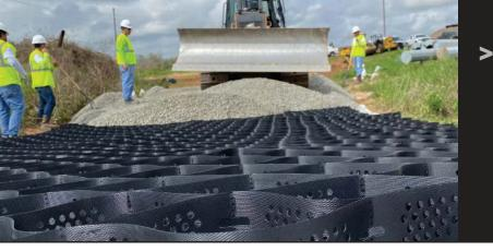
BaseLok<sup>™</sup> GeoCell is a confinement system that performs better than conventional crushed stone sections, and it provides an expedient construction technique for access roads over soft ground without being adversely affected by wet weather conditions.
